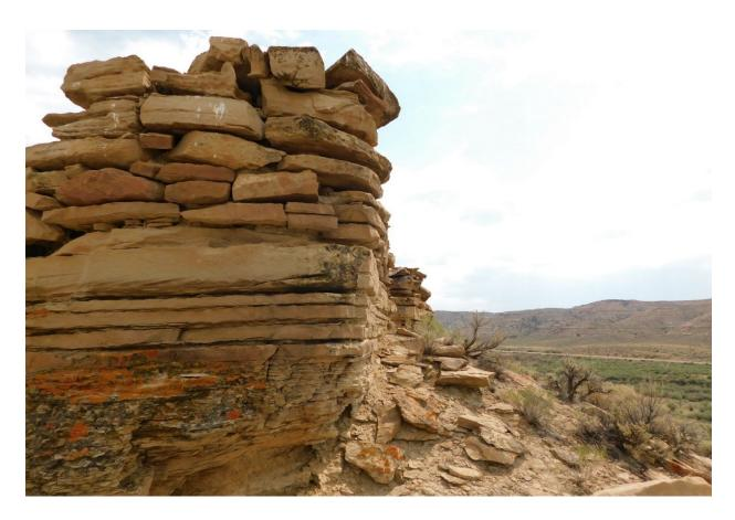
Figure 48. Image of exemplary flush walls at Rocky Ford. Any billowing seen here is a probable necessity for balance. Facing southwest. Summer 2021. Photograph by Joshua Bauer.
