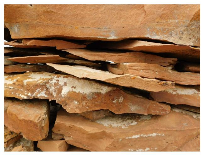
Figure 45. Detail of dry-laid masonry work at Mountain, characteristic of most of the pinnacles. Careful attention was needed to achieve balance and uniformity. The thinner slabs used at this site are also on display here. Summer 2021. Photograph by Joshua Bauer.
