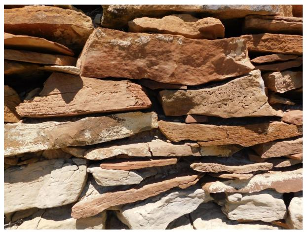
Figure 41. Detail of south wall at Edge, showing sandstone slabs in their natural state. No rocks appear to have been shaped at any of the sites. Instead, stacking was carefully arranged according to dictates of natural forms. Summer 2021. Photograph by Joshua Bauer.
