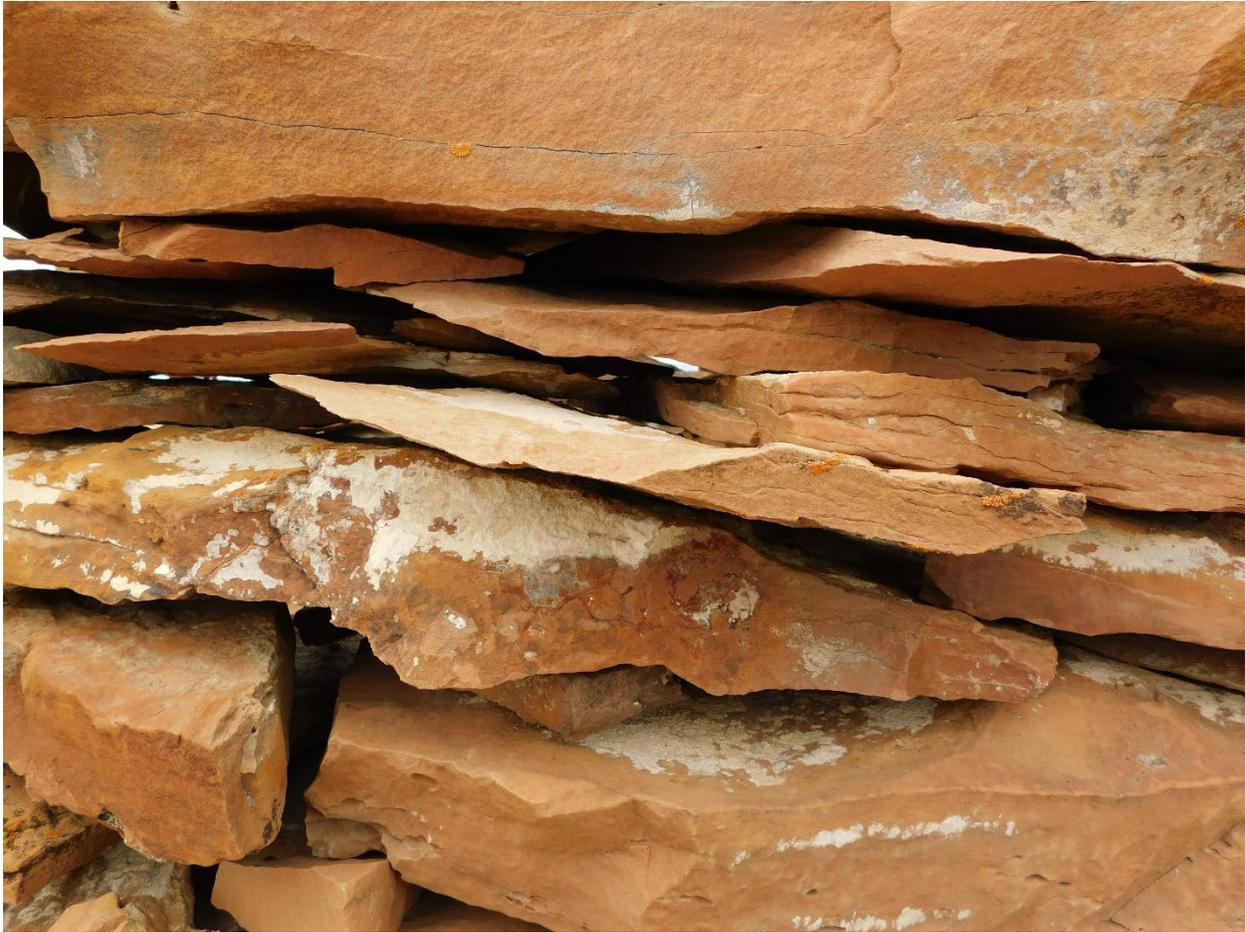
Figure 45. Detail of dry-laid masonry work at Mountain, characteristic of most of the pinnacles. Careful attention was needed to achieve balance and uniformity. The thinner slabs used at this site are also on display here. Summer 2021. Photograph by Joshua Bauer.
