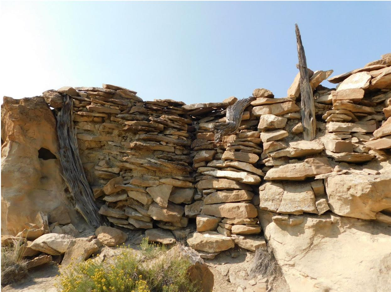
Figure 50. Showing north wall at Texas Creek, where frequent billowing is a function of building such high walls. This photo also shows the juniper posts embedded in wall as reinforcement or as roof elements. Facing north. Summer 2021. Photograph by Joshua Bauer.
