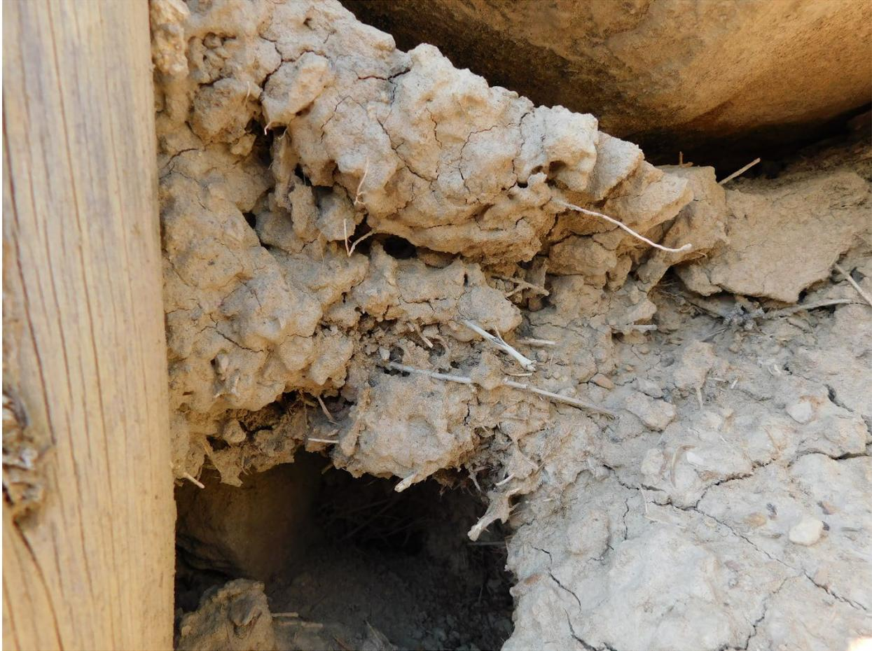
Figure 44. Showing fibrous temper of sticks, roots, and grass added to the mortar in Texas Creek's north wall. Summer 2021. Photograph by Joshua Bauer.
