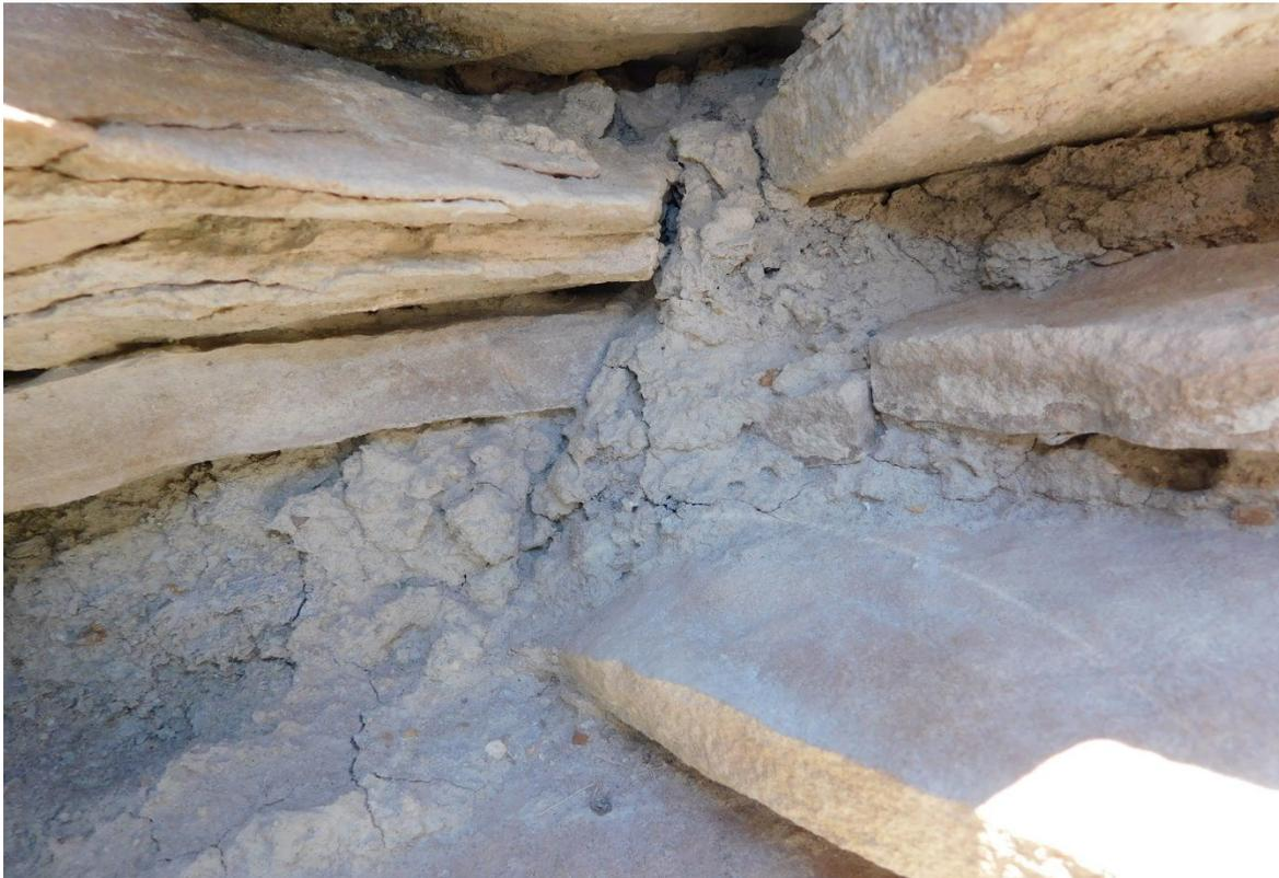
Figure 43. Detail of mortar used at Edge, composed of a light brown silt loam and a crushed sandstone grit aggregate. The same paste was used at Rocky Ford. Summer 2021. Photograph by Joshua Bauer.
