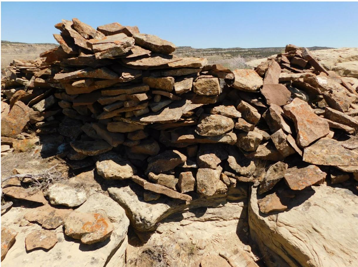
Figure 51. Showing a relatively intact portion of Spook Mountain, where extensive billowing attests to rushed work more so than necessity for structural integrity. Facing south. Summer 2021. Photograph by Joshua Bauer.
