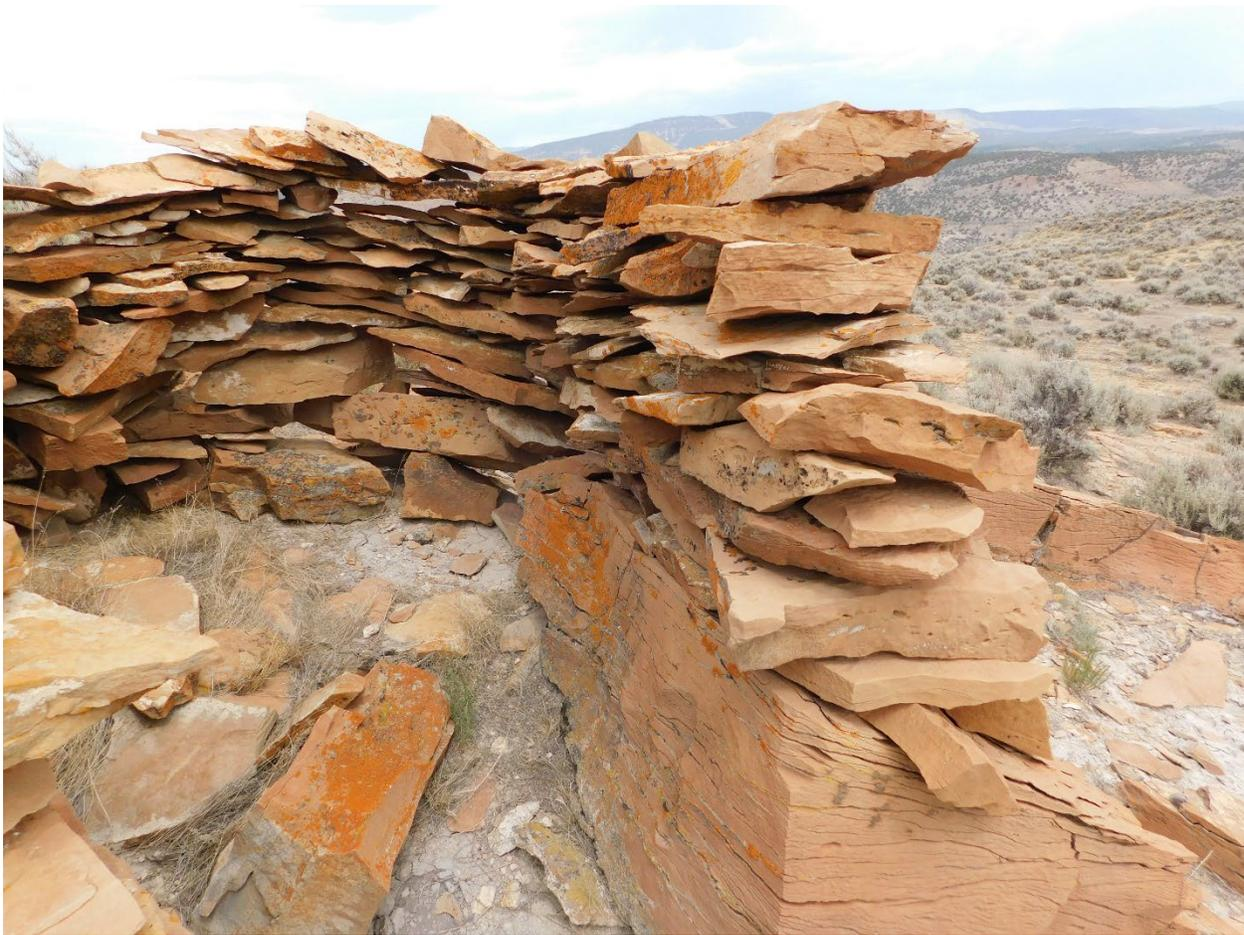
Figure 49. Showing flush walls at Mountain, where tapering appears to be a design feature that the builders used for balance. Facing east. Summer 2021. Photograph by Joshua Bauer.
