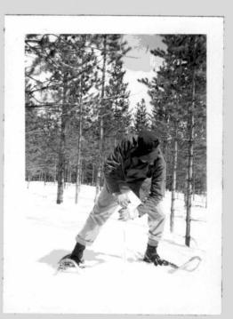
Figure Five - After the snow tube touches the surface of the ground, the tube is rotated to force a plug of soil into the cutter.
