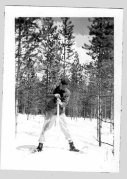
Figure Four - The snow tube is held vertically and is forced into the snow pack smoothly and steadily.
