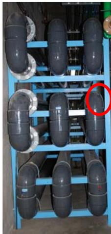
Figure 11 - Intermediate Sampling Point
