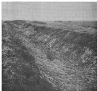
Dry and cracked loessial materials Initial Stage in sediment ponding. in lateral bottom before sedimenting. (Note wetted fringe.)
