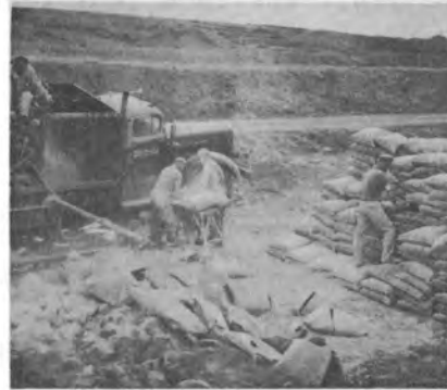
View of hopper where bentonite and dispersant was added to water.
