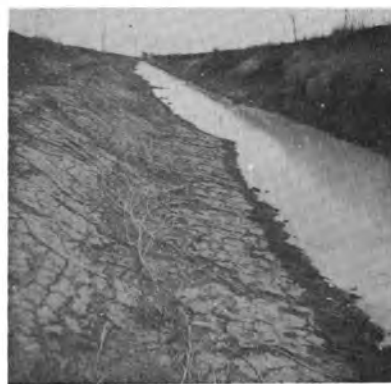
Dry and cracked loessial materials Initial Stage in sediment ponding. in lateral bottom before sedimenting. (Note wetted fringe.)
