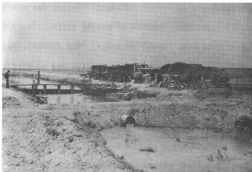
Equipment set-up for mixing. Temporary holding pit constructed so that mixing could be completed. Pump on left used for supplemental jetting.
