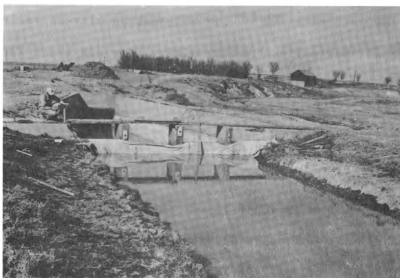
Initial filling of pond at Mile 11.0. Note canvas for water-proofing and mixture testing by man on structure.
