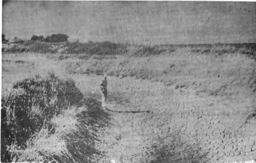
Natural sediment cake in canal as a result of muddy irrigation water. Cracks were formed during a two-week period after water was shut off in Superior Canal -- Bostwick Unit, Nebraska and Kansas.
