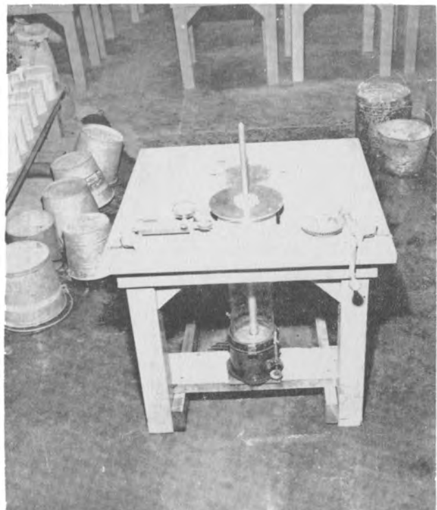
Vane Borer apparatus for determining cohesion.
