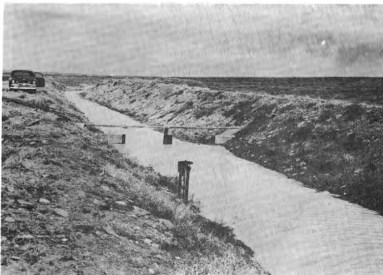
Existing check structures utilized for ponding the mixture. Ponding interval was about 6 to 10 hours. May 7, 1953
