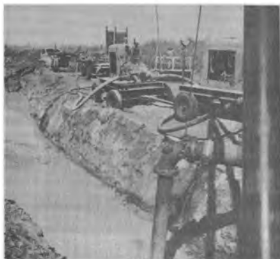
View of discharge line from jet, and holding pit and equipment.
