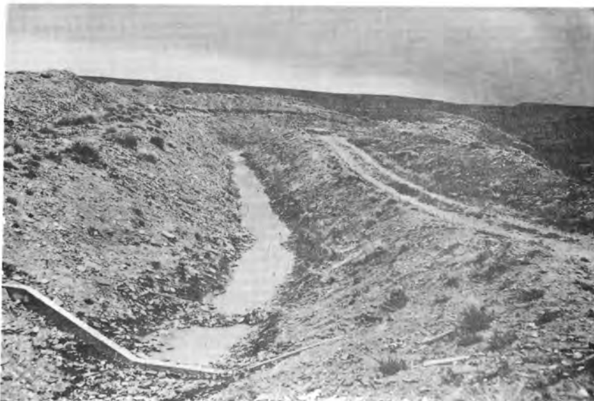
Clear water remained in low sections of lateral for about a week after the sedimenting. Before treatment, the lateral dried up within a day or so. May 15, 1953
