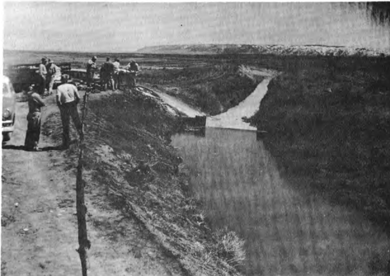
Bentonite slurry mixing operation for initial sedimenting experiment. Slurry being diluted by flow of clear water over weir(Sta 2+56, lat 218). May 6, 1953
