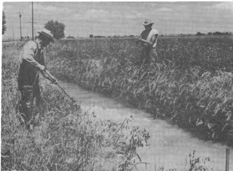
Mixing operation by air jetting into wet bentonite layer on lateral bottom, Lateral No. 4 near Wellington, Colorado.
