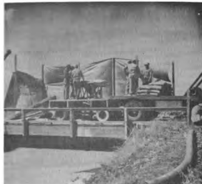
Bentonite being unloaded directly from truck into jet hopper.
