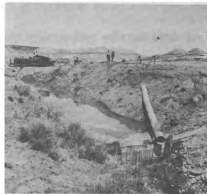
View of slurry addition point. Diluting flow released over weir.
