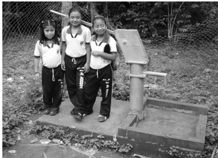
Figure 4.7 EWB installed school well The school well pictured above is the new well in the right portion of the air photo. This well was placed at the lowest topographic point in the community along a visible, but dry channel bed.
