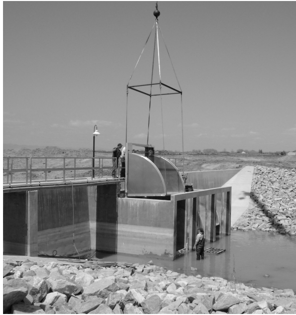
Figure 2. One of three gates on the Greeley #2 canal is re-installed during the spring of 2007 following a repair that was accomplished over the winter when the canal was out of operation.
