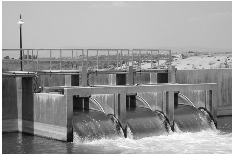
Figure 3. Three gates operated concurrently can handle the 600 CFS flow delivered from the Kern Reservoir which is an equalizer on the Greeley #2 Canal.
