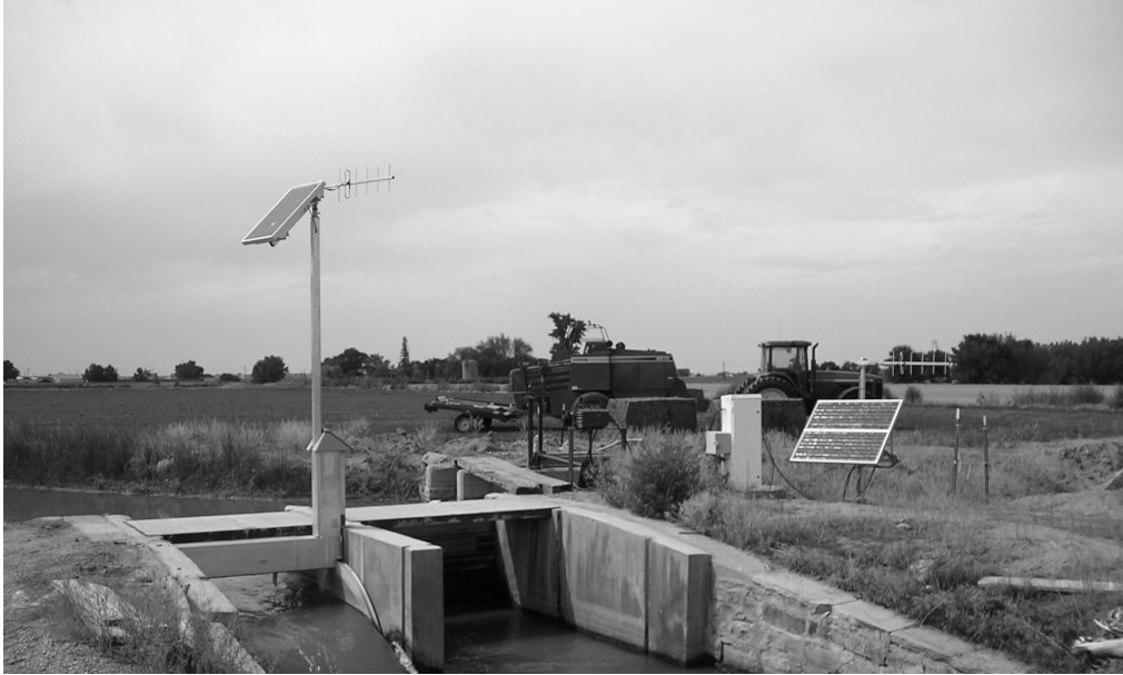
Figure 4. A bifurcation in the Greeley #2 has historically been used to move storm flows down preferred reaches of the canal and to serve as a place to waste excess flows back to the river in order to avoid a breach of the canal. The photograph shows a Rubicon gate used to hold deliveries on a portion of the canal. A radial gate on the other leg of this bifurcation can be opened to release storm flows.
