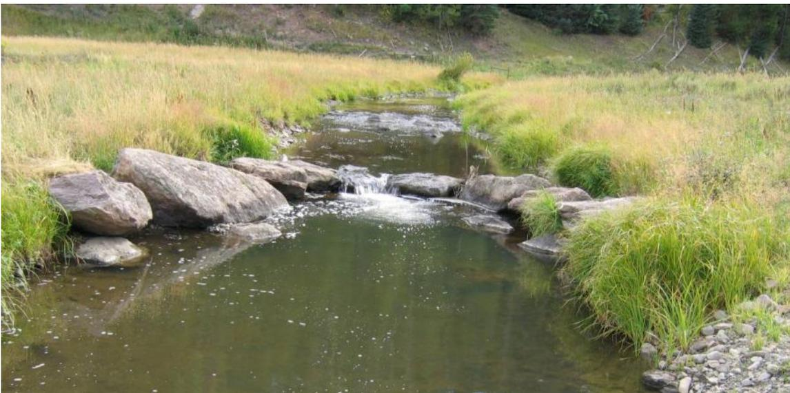
Figure 3.8 – U-weir on South Fork Little Snake River at low flow.
