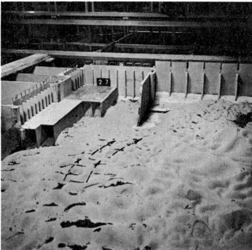
Fig. 22. Extension of tunnels 1 and 2 only. Tunnel No. 2 is set back 40 ft from the end of Tunnel 1. Tunnel 1 is even with the end of the T-S head regulator.
