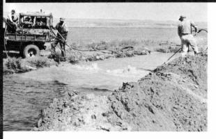
Dilute the thick slurry (usually 6 to 8%) with the clear water from the by-pass. Add your slurry into the
