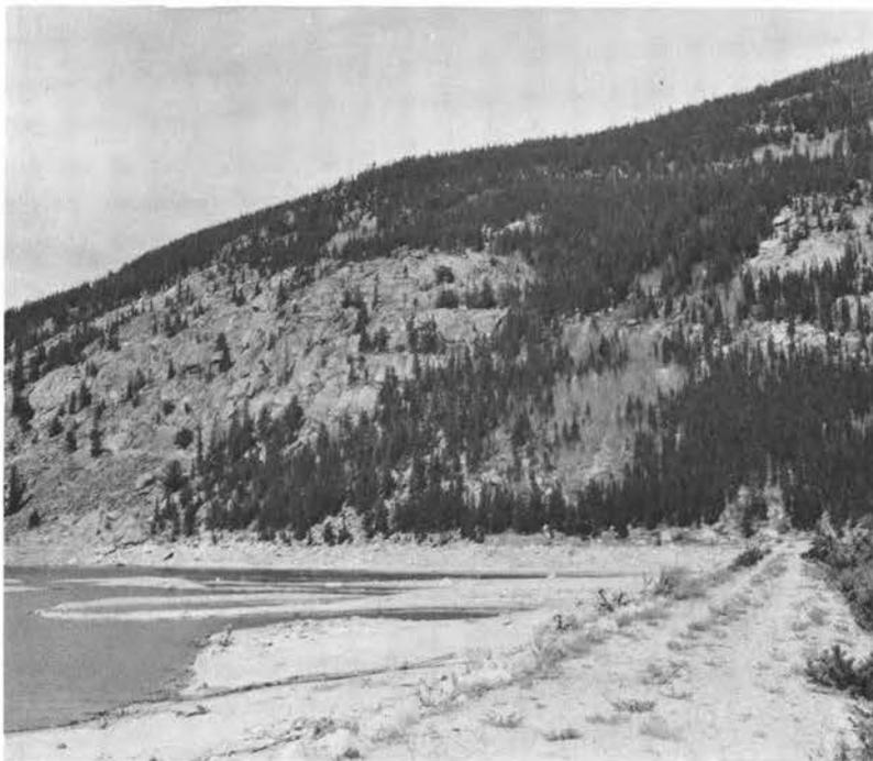
Figure 3. The coarse gravel dam which forms Comanche Reservoir.
