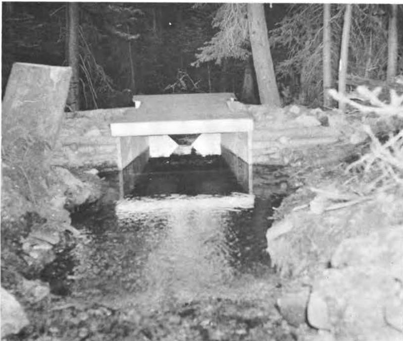
Figure 29. The Upper Little Beaver stream gaging station. The v-notch weir used to measure low flows is in place. The view is downstream.
