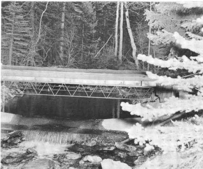
Figure 31. The Lower Little Beaver stream gaging station showing the broadcrested weir used as a control.
