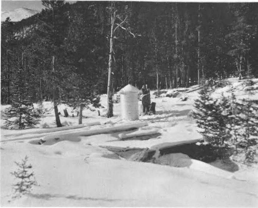
Figure 32. Fall Creek gaging station. The natural control is covered and heated to prevent icing.
