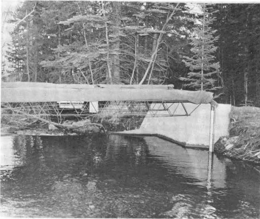
Figure 30. The Lower Little Beaver stream gaging station. Note the cover and heater used to prevent icing of the control section. The view is downstream.
