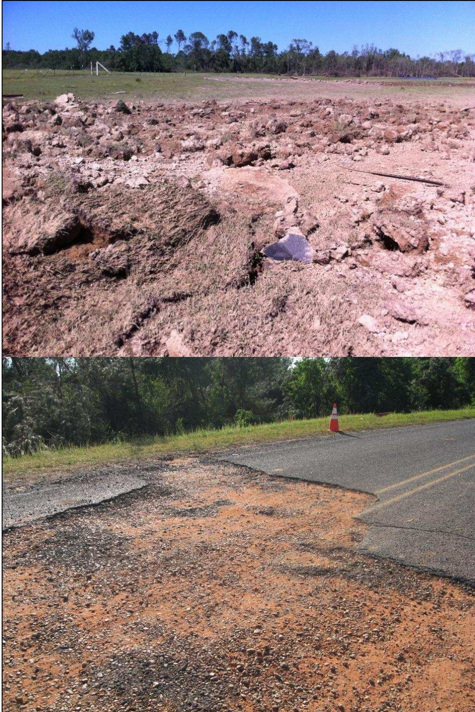
**Figure 5.2:** Image of ground (top) and road (bottom) scouring from the Philadelphia-Kemper, MS EF5 tornado. Image courtesy of the Jackson, MS NWS Office (NWS JAN 2011).
