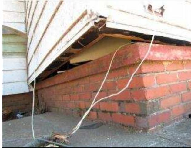
**Figure 1.6:** Overturning failure of a residential structure during the April 27, 2011 tornado in Tuscaloosa, AL.
