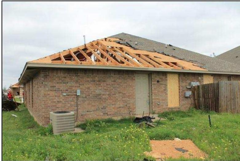
**Figure 1.2:** Failure of roof sheathing during the May 20, 2013 Moore, OK tornado. The remainder of the home performed well.
