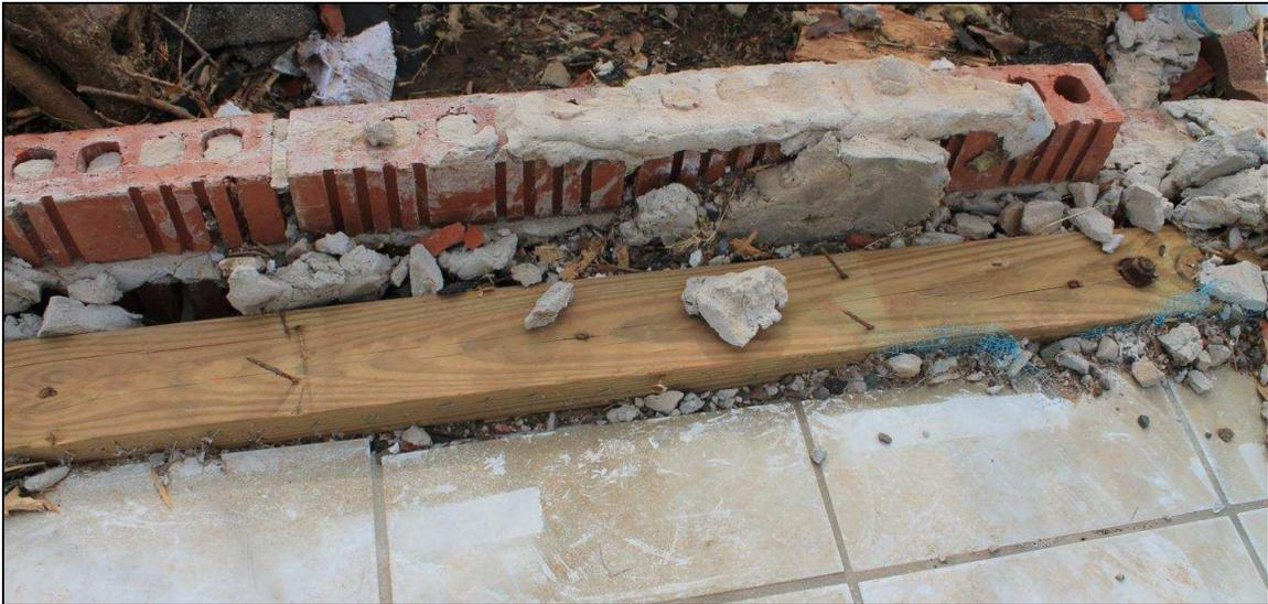
**Figure 1.7:** Failure of the wall-to-foundation connection due to wall stud pull-out. Note the bottom plate is still attached to the foundation and the nails to the wall studs remain in place.
