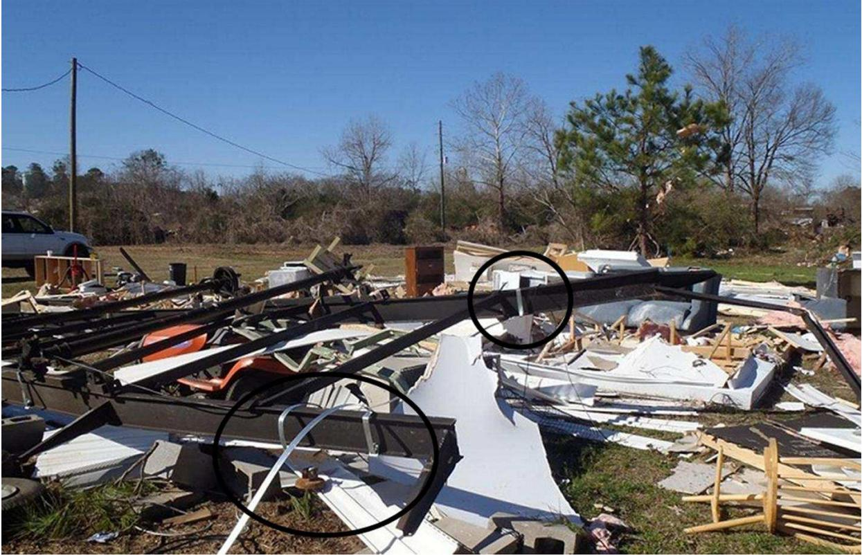
**Figure 5.5:** Catastrophic damage to a manufactured home from an EF2 tornado in Perry County, Alabama. Tie-downs are indicated in the black circles.
