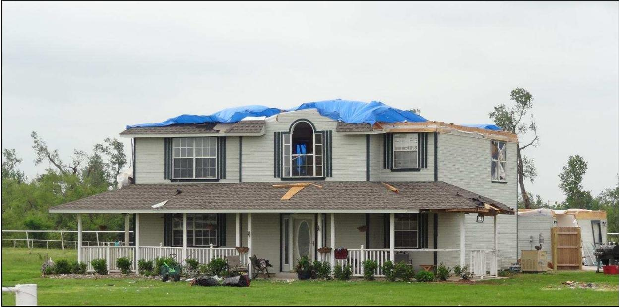
**Figure 1.4:** Failure of the roof-to-wall connection at a home during the May 20, 2013 Moore, OK tornado.
