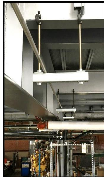
**Figure B-6.** Picture showing tubing supported along the overhead by clamping to I-beams.
