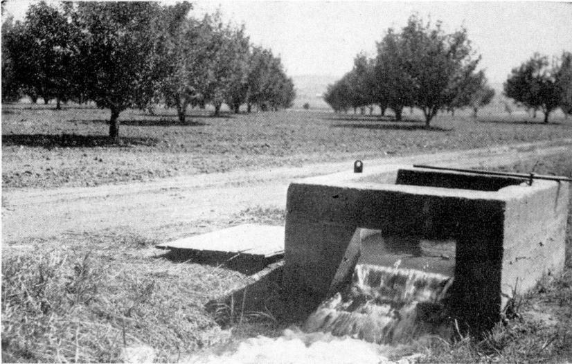
Riser and measuring weir combined, on an underground ditch system.
