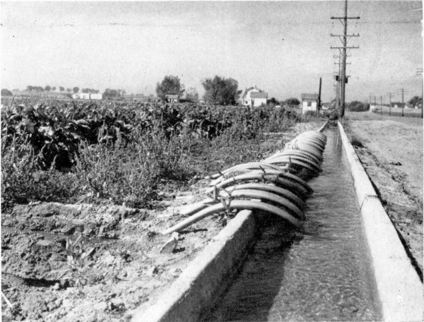
Aluminum siphon tubes operating in a concrete-lined lateral provide even distribution of water to a maturing sugar beet crop.
