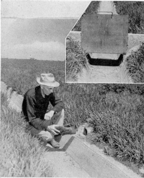
The sunken type of field lateral, concrete lined with checks to raise water to permanent spiles. Wooden plugs wrapped with burlap or an old potato sack are used for spill plugs when needed. The banks are planted to bromegrass to stabilize them and to eliminate most weeds.
