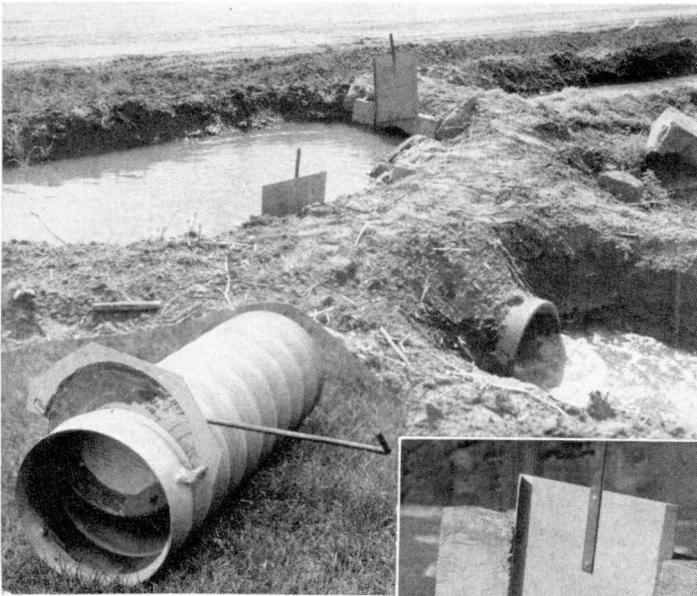
The two gates (upper center) are steel sheets installed in pre-cast concrete head walls attached to lengths of concrete pipe. In the left center is a quick-opening and closing steel gate built into a short length of corrugated steel pipe. At the right is a steel gate installed in a precast head wall and tube.
