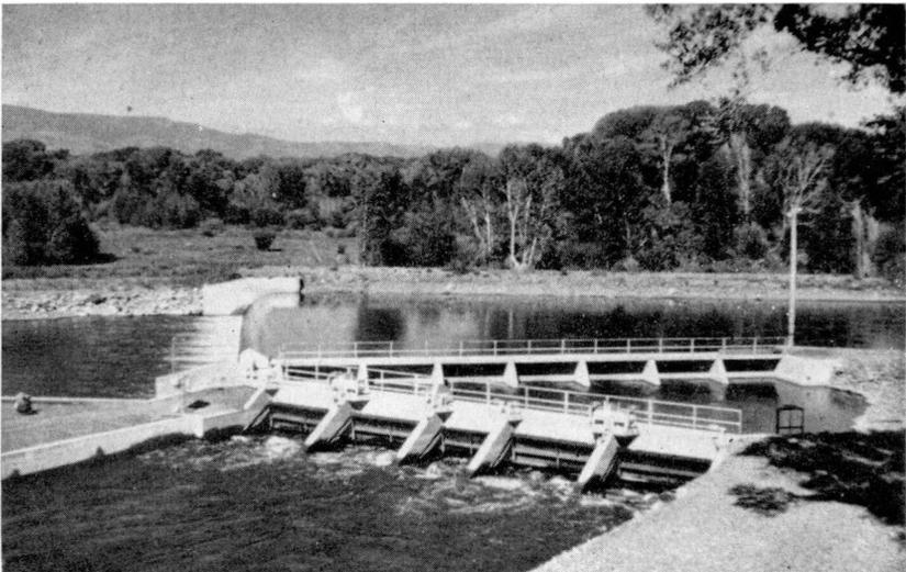
One of the larger canal diversions in Colorado. Automatic electrically controlled head gates of the Rio Grande Canal, mutually owned and operated, Del Norte, Colorado.
