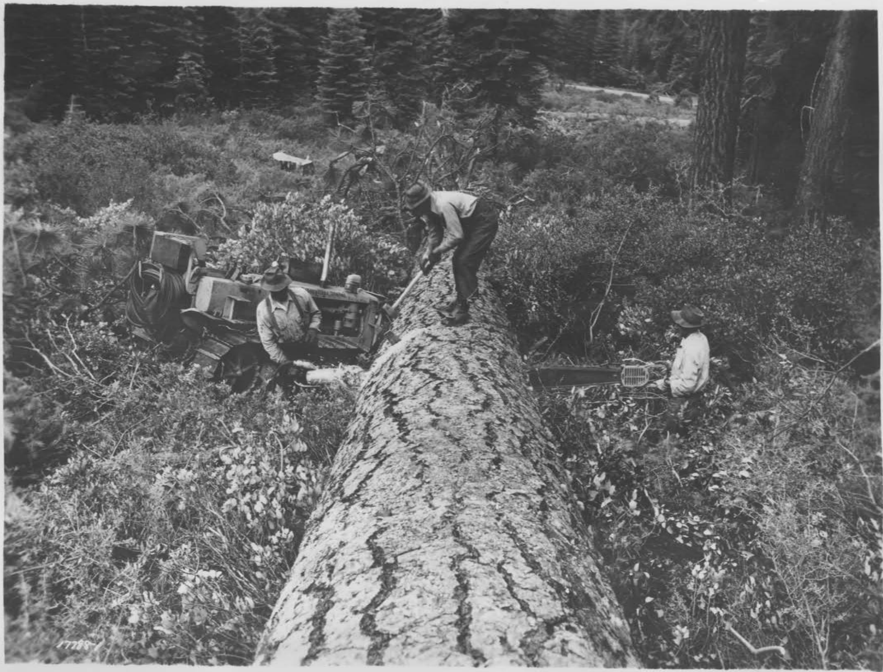
Plate VIII: Bucking with Atkins electric power saw.
