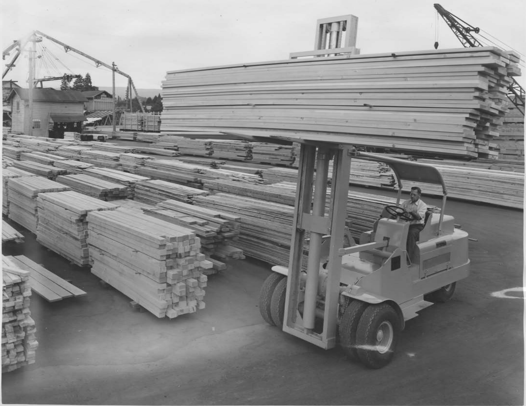
Plate XVII: Elevating lumber into position for piling with lift truck.
