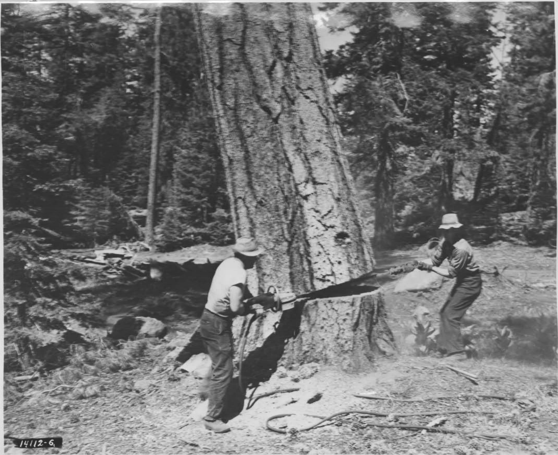
Plate VII: Felling with Atkins electric power saw.
