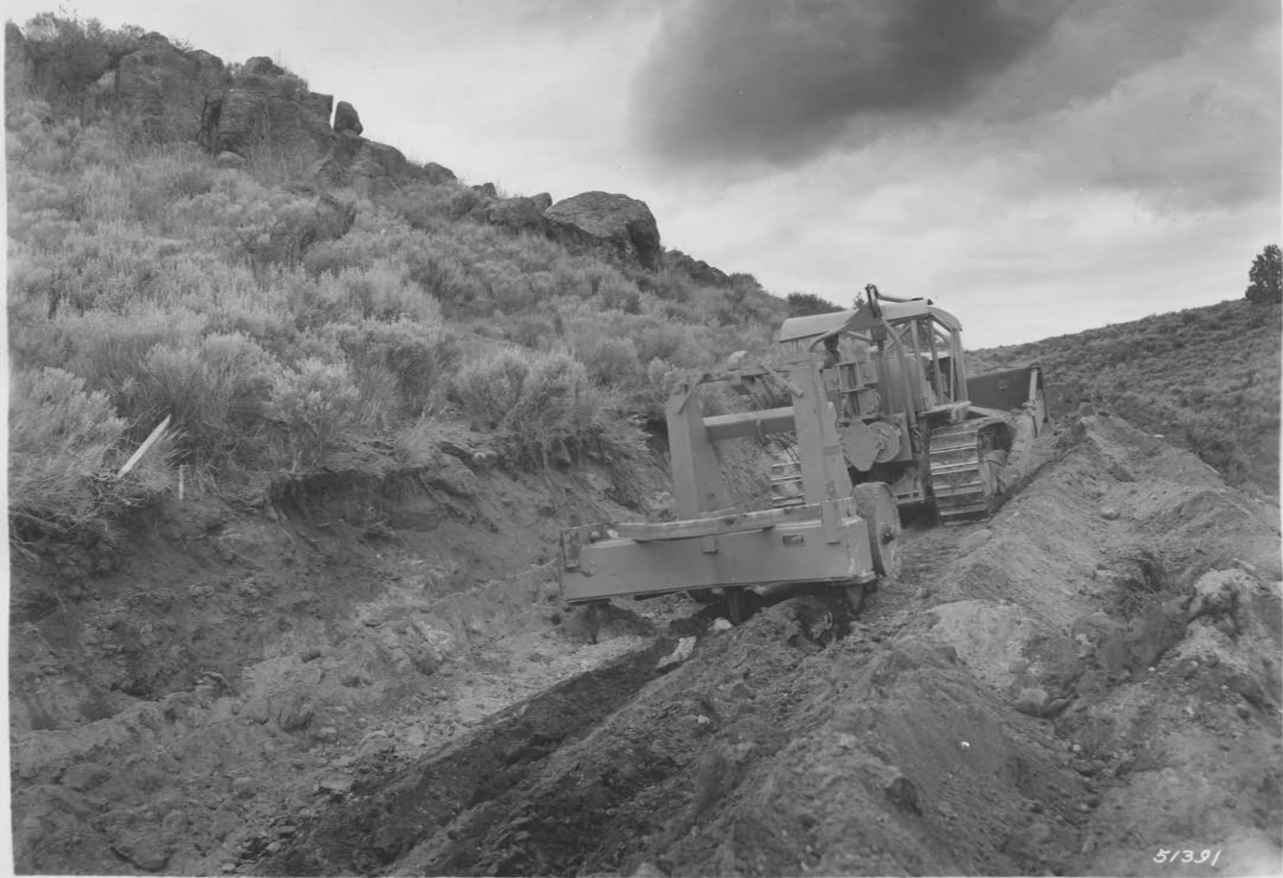
Plate II: Root pulling with Caterpillar tractor.
