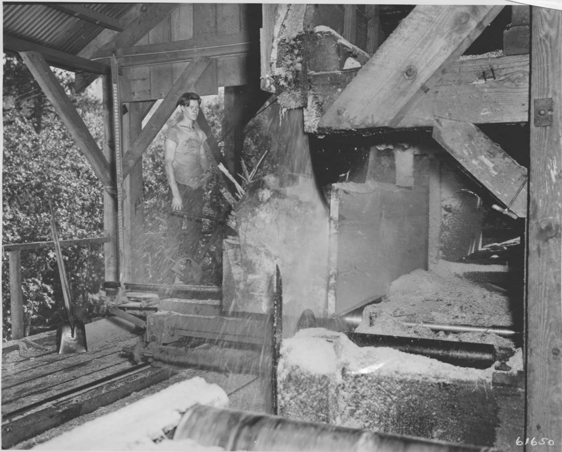
Plate XV: Sawing lumber with double circular head saw.
