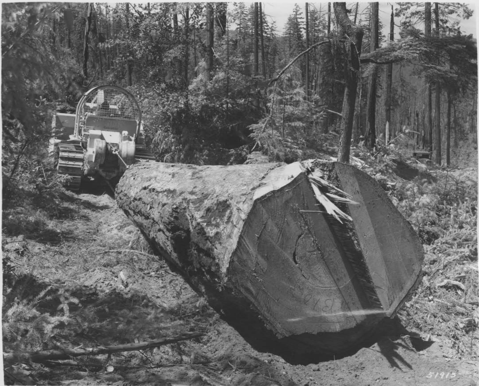
Plate X: Ground skidding with Caterpillar tractor.
