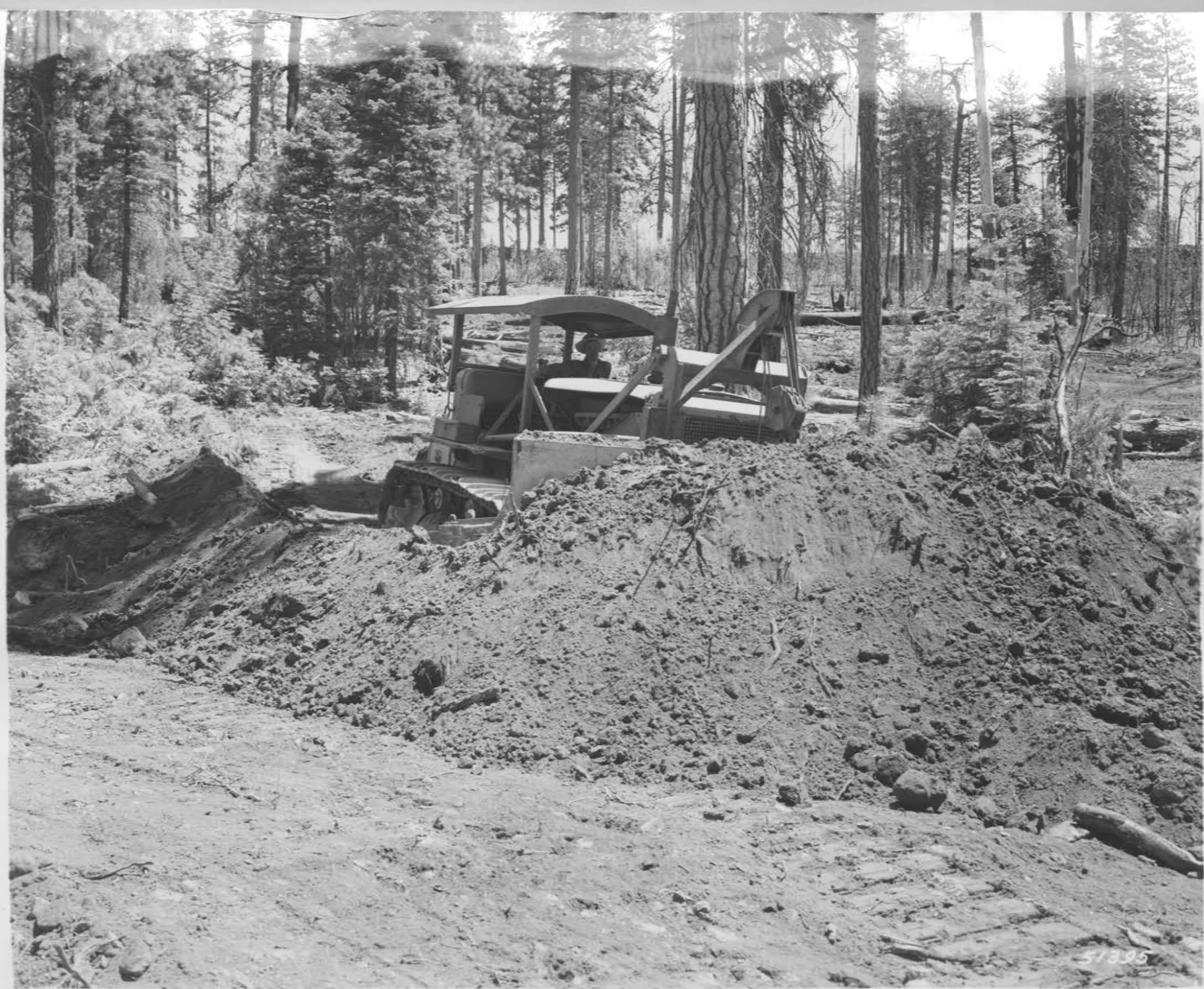
Plate III: Road grading with Caterpillar tractor.
