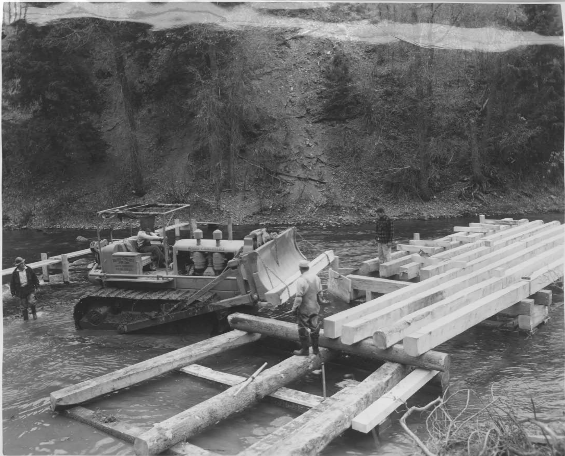
Plate V: Tractor positioning bridge timbers.
