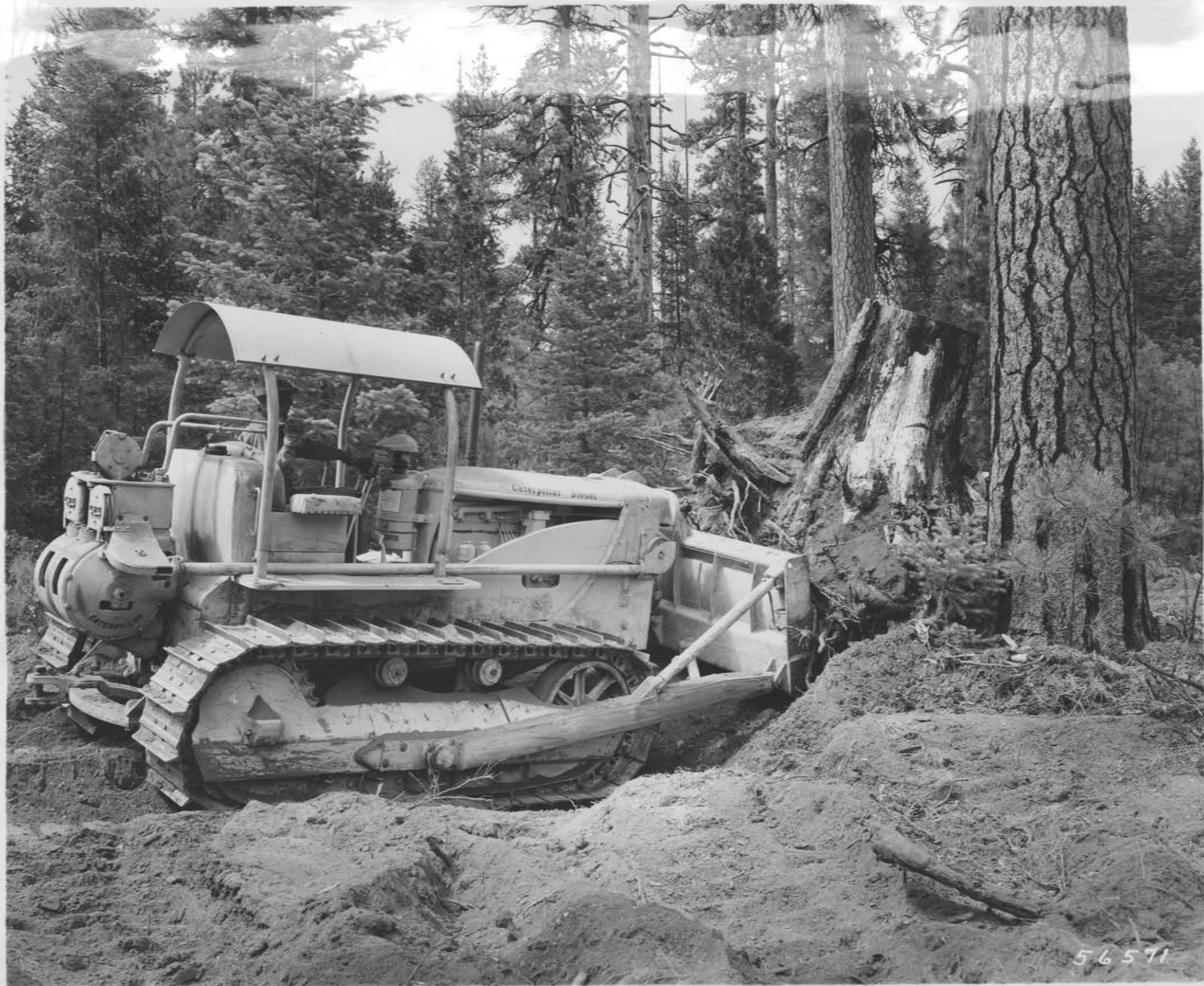
Plate I: Road clearing with Caterpillar tractor.
