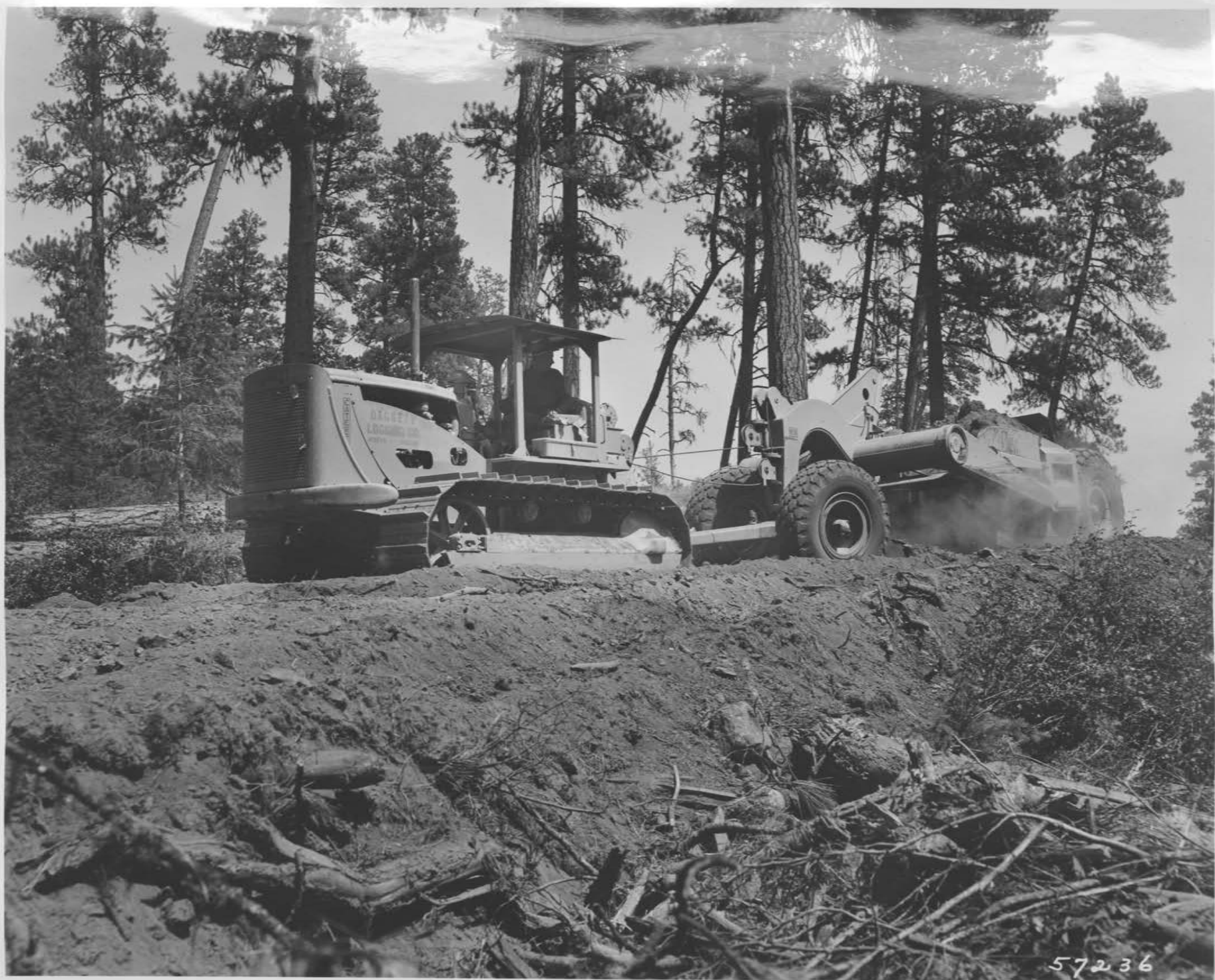
Plate IV: Tractor and carryall moving dirt for road construction.
