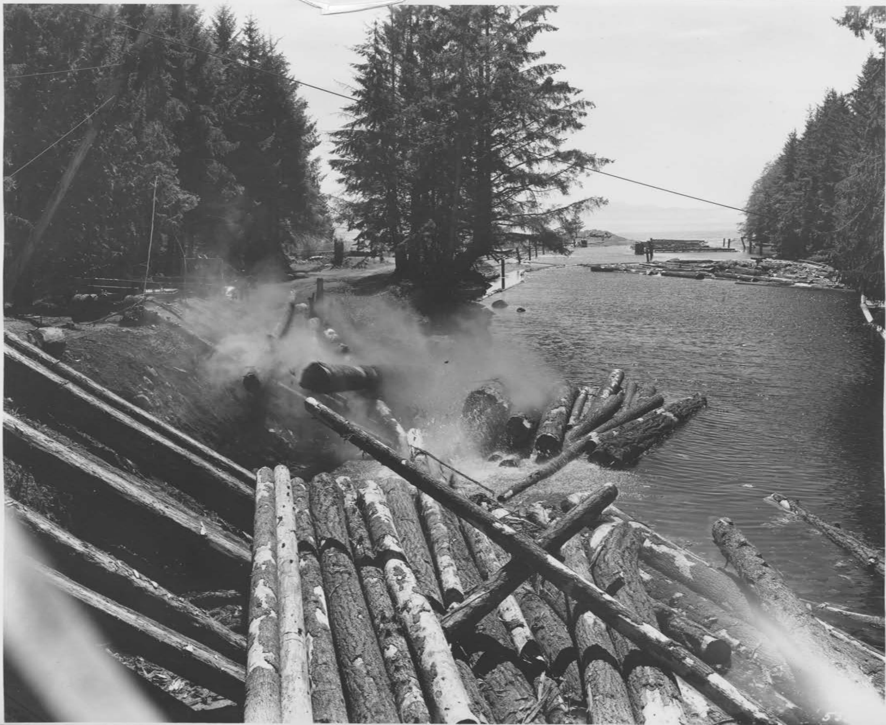
Plate XIII: Unloading with Gin pole and bridle.
