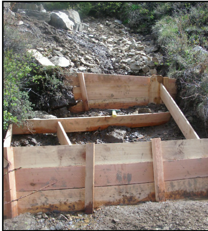
Figure 2. Front view of plank walls used to stabilize fill material for recontouring gullies. Prior to backfilling and revegetation on Mt. Massive, 2004.
