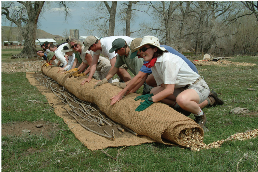
Volunteers complete a homemade "biolog" to stabilize the banks of Left Hand Creek.
