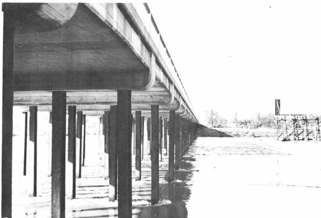
Forest of piling under East Sand Slough Bridge at Red Bluff.
