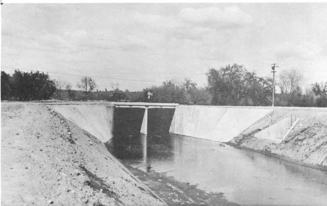
Stream lining of double-box culvert with warped wingwalls and half-round nosing.
