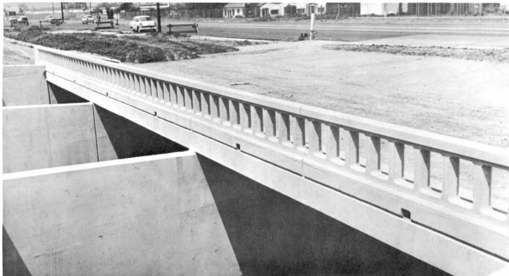
Web walls between parallel bridges over San Francisquito Creek at Palo Alto
