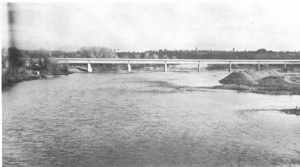
Varied-skew piers on skew-curved bridge over Sacramento River at Redding (see Fig. 3).
