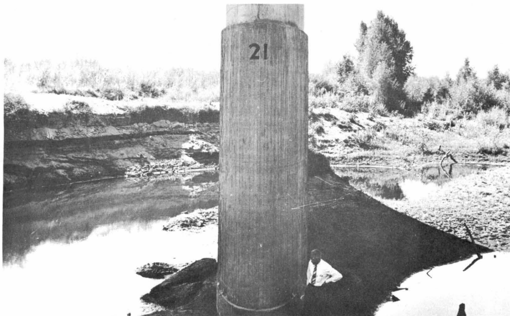
Scour around Pier 21 of Feather River Bridge at Yuba City due to cross current in overflow channel.
