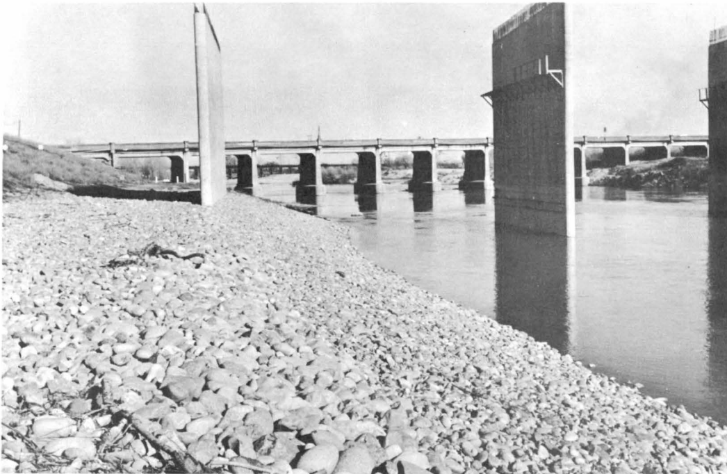
New thin-wall piers of Yuba River Bridge at Marysville compared to massive piers of old bridge
