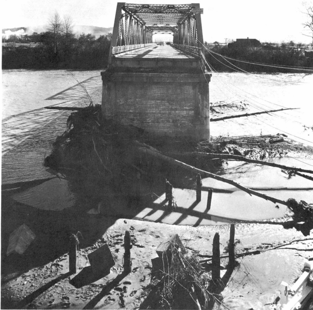
Drift on abutment pier of Mad River Bridge near Arcata; pile-trestle approach destroyed by drift.
