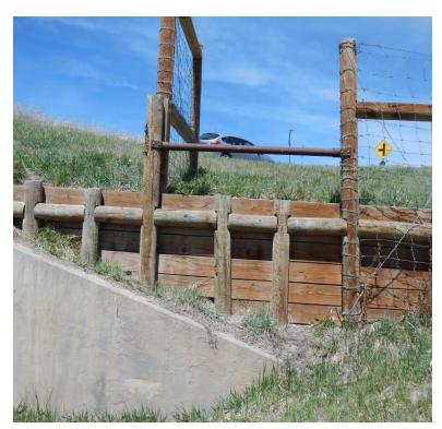
Figure 17. Dry Creek escape jump along Highway 550 from the creek bed.
