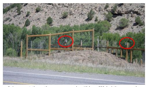
Figure 2. A representative earthen escape ramp along Highway 550 depicting camera placement (cameras circled in red).
