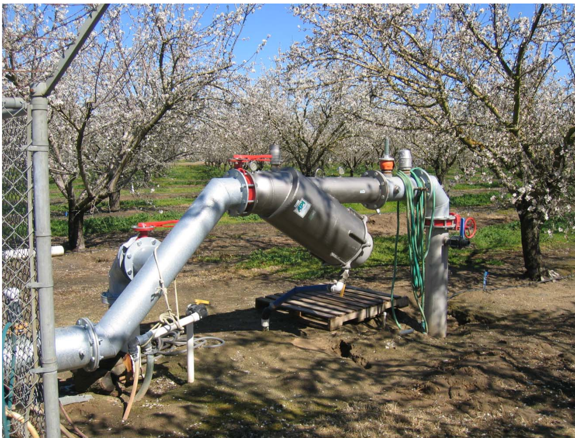
950-GPM Filter Connected to Both A Well and TID Water
