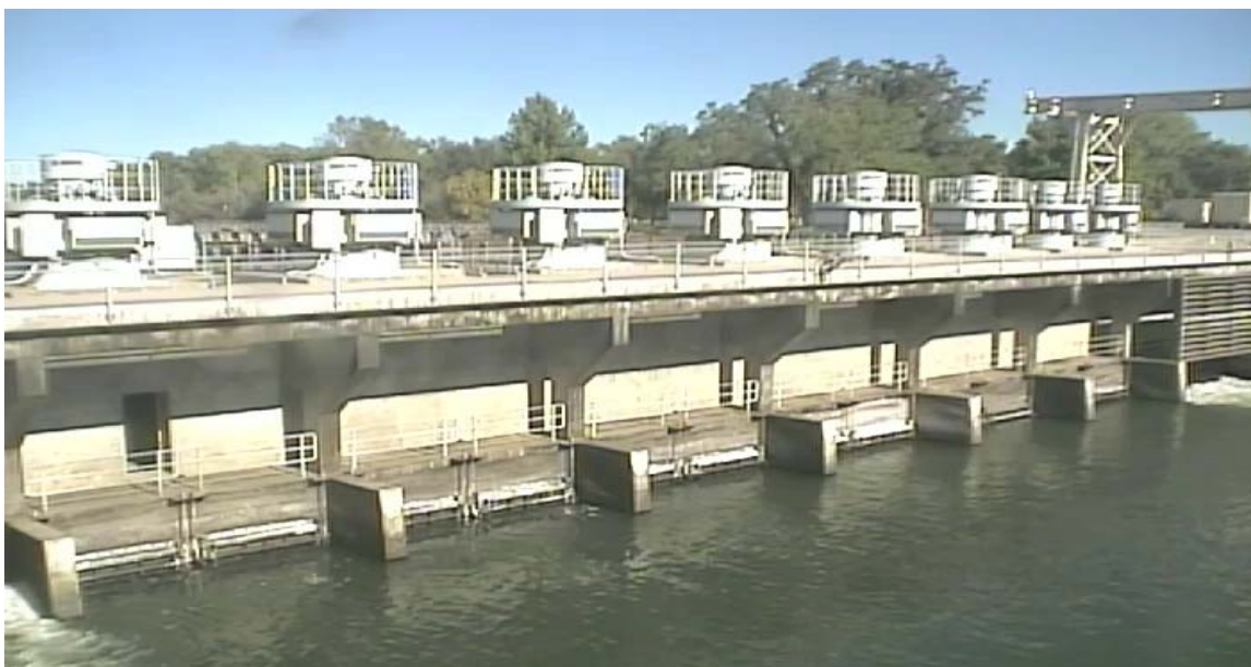
Figure 2. GCID's main pump station, located on the Sacramento River, has the capability of pumping 3,000 cubic feet per second (cfs). SCADA allows canal operators to make pump changes remotely, monitor water elevations, and measure the water quality entering the District's main canal.
