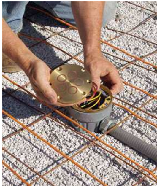
Figure 1.6 Snow sensor installation in electric system [17]
