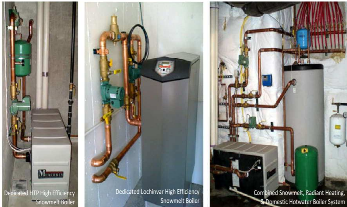
Figure 2.3 Typical snowmelt boiler systems [24]
