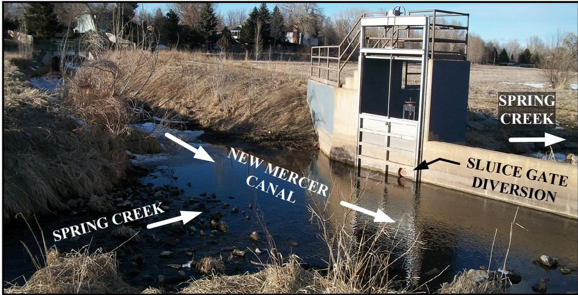
**Figure 3-7: Confluence of flow at Spring Creek and New Mercer Canal. Flow comingles in the New Mercer Canal before being discharged to Spring Creek via a sluice gate.**
