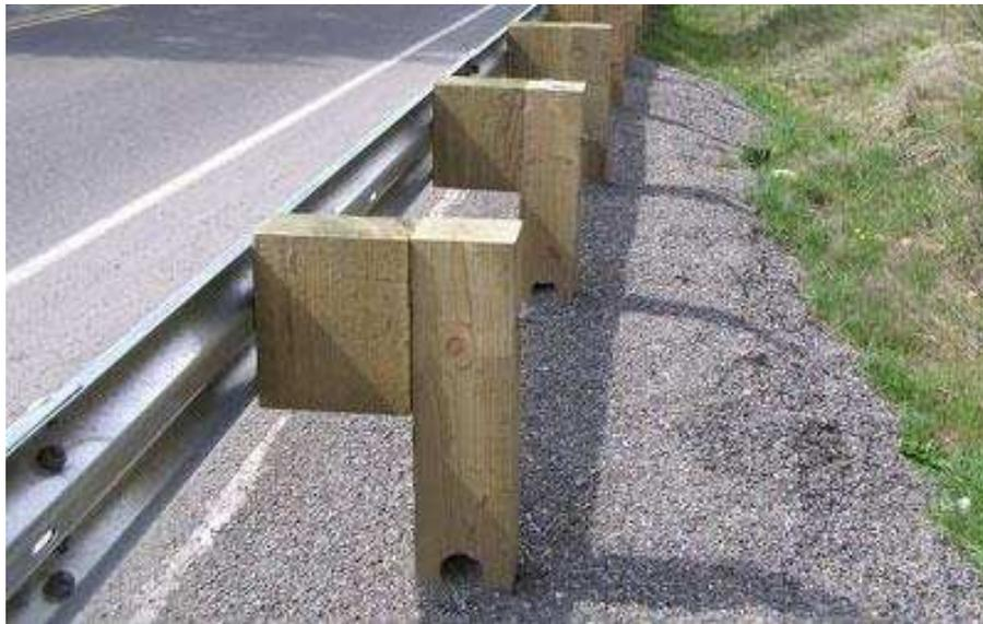
**Figure 5: Semi-Rigid Barrier System: Strong Post W-Beam (Source: [safety.fhwa.dot.gov](http://safety.fhwa.dot.gov))**
