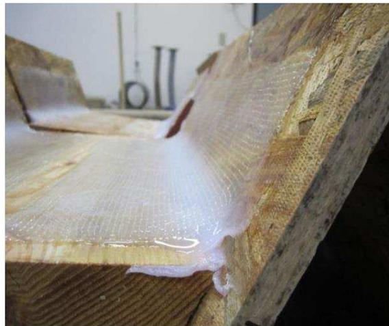
**Figure 3 – Wood Preparation Close-up (Source: Fyfe)**
