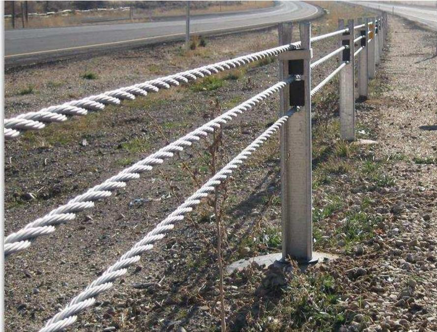
**Figure 4: Flexible Barrier System: Three-Strand Cable (Source: [blog.udot.utah.gov](http://blog.udot.utah.gov))**
