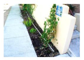
Figure 2: Drip Irrigation Utilizing Graywater
