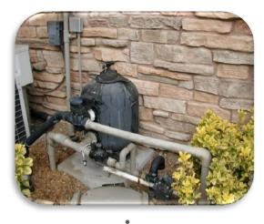
Figure 3: ReWater Graywater Reuse System for Irrigation using a sand filter
