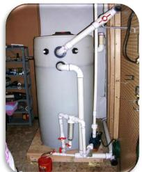
Figure 4: Storage Tank for Subsurface Irrigation Graywater System
