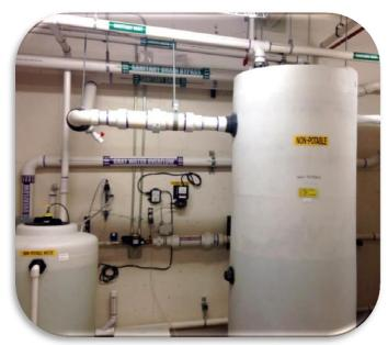
Figure 3: Graywater Reuse System for Toilet Flushing in Aspen Hall at Colorado State University
