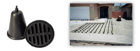
Figure 6: ReWater emitters (left) and emitters being installed under turf lawn for subsurface irrigation (Rewater<sup>®</sup>, 2014 Link)
