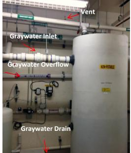
Figure 5: Graywater Tank and Components
