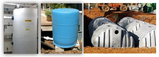
Figure 3: Photograph (left to right) Indoor, outdoor, and underground storage tanks (Bergdolt, 2011 URL: Link)
