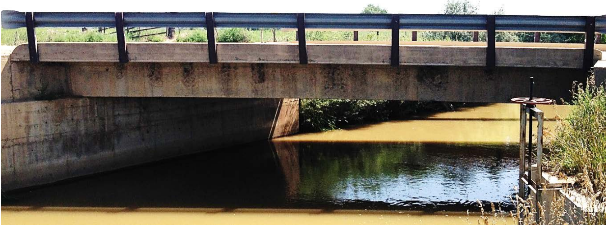
Figure 8.1 Bridge LR3-0.2-50 east elevation view
