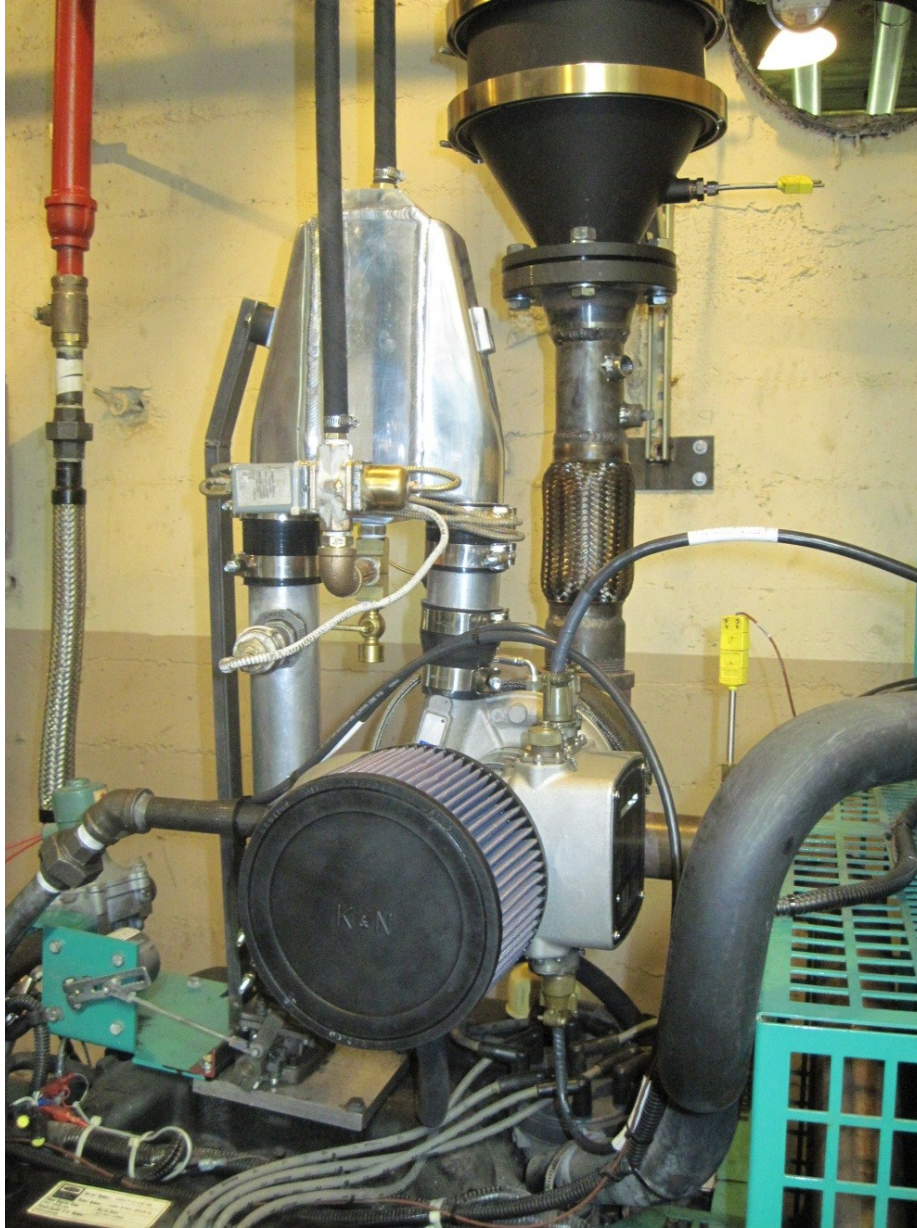
Figure 3-5: Intercooler installed and plumbed for air and water
