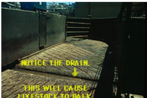
**Drains should be located outside of the areas where animals walk. A drain or a metal plate running across an alley will cause balking.**
