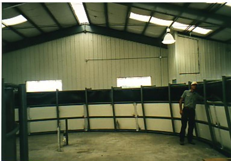
Well designed curved single file chute with solid sides to block the animal's vision. White translucent skylights provide good lighting with no shadows. The black strip along the top of the chute (race) is flexible rubber conveyor belting. The belting blocks the animal's vision and handlers can easily reach under the belting to move cattle.
